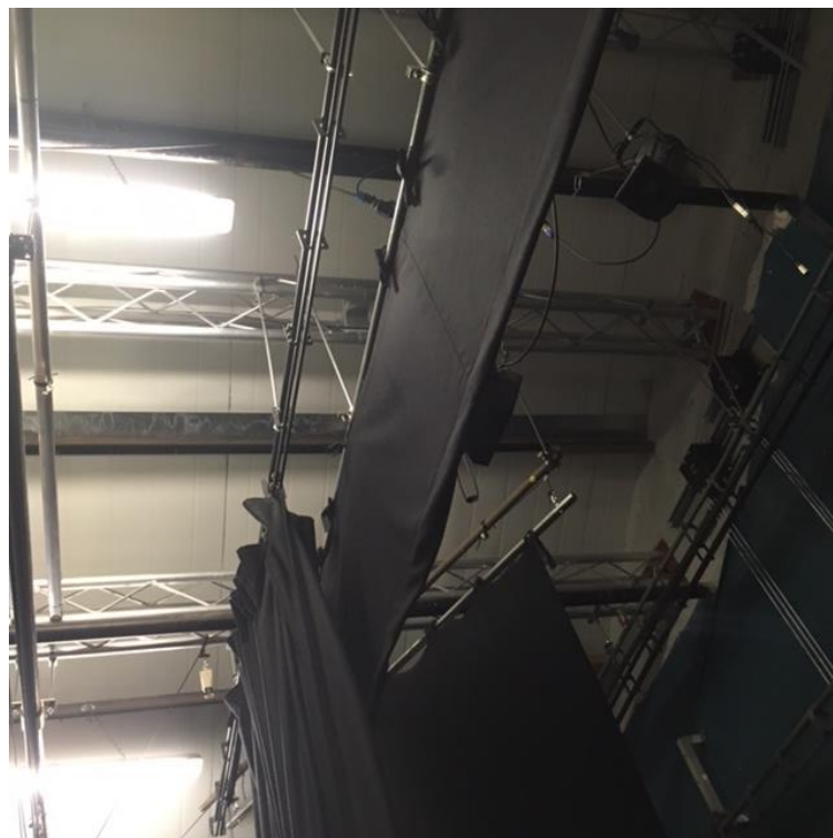
Figure A1.4 – underside of roof as viewed from the stage
