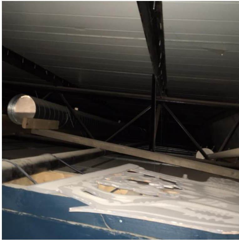
Figure A1.3 – ceiling void above main hall area
