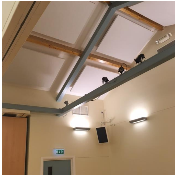
Figure A1.9 – Studio underside of roof – note acoustic panels
