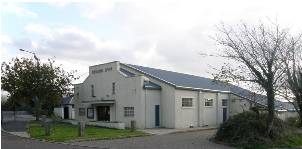
Re roofed revitalised with a small annex
